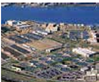
4 Blue Plains Wastewater Treatment Plant, Washington, D.C.
