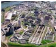
3 Overflow Abatement Program, Nashville, Tennessee
