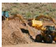
14 Metropolitan Government of Nashville and Davidson County/Overflow Abatement Program
